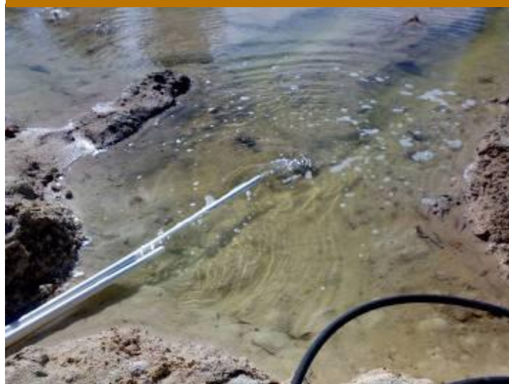
Photo 8: Airlifted water entering the nutrient trench.
