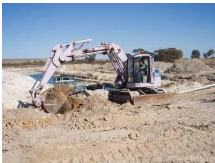
Photos 1 and 2. Above: excavating the trench, and below the trench ready for cages.
