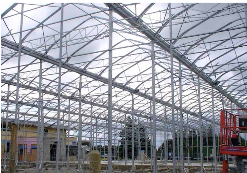
Framework for CA$18 million R&D unit
