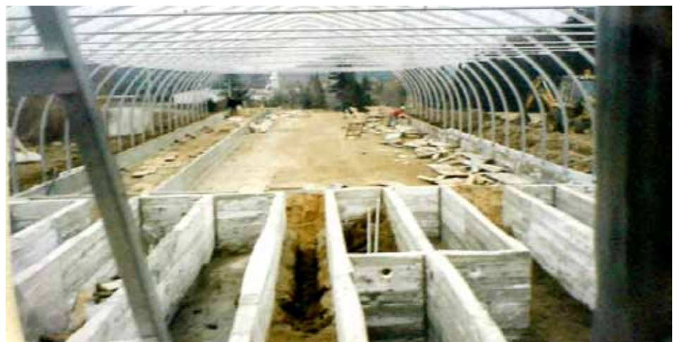
Concrete skeleton of production area
