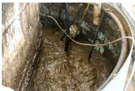
Solids waste digestion
